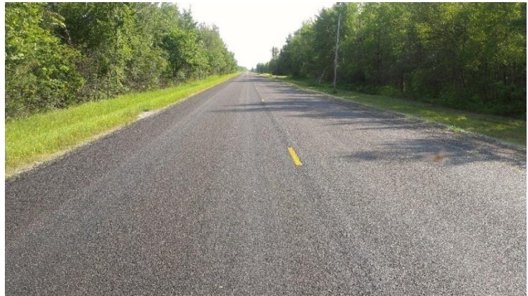
Figure 2 - TH 89 after Placement of Chip Seal
