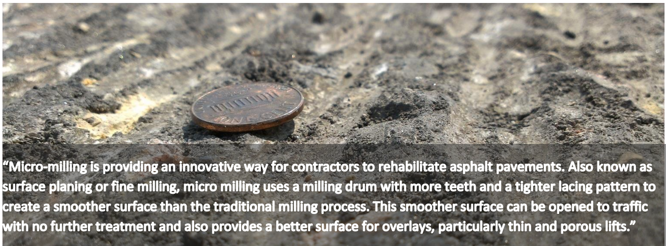
Figure 1 – Finished Micro Mill Texture of TH 89
